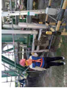
Measure flammable atmospheres before starting hot work.
