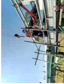
Working at height used safety harness and hanging while work.
