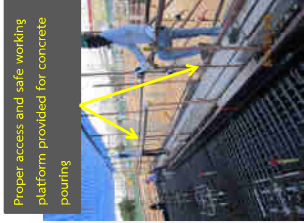
Handrail was erected to prevent workers from falling
