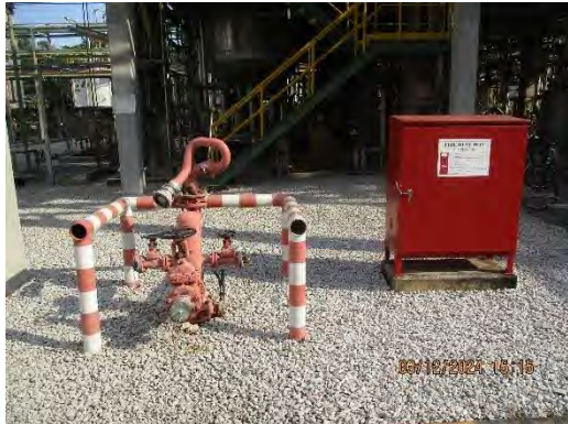
Water Hydrant/Fix Monitor
