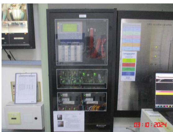
Fire alarm control panel
