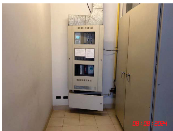
Fire Alarm Control Panel
