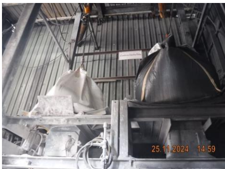
Hydrate Lime & Activated Carbon Injection
