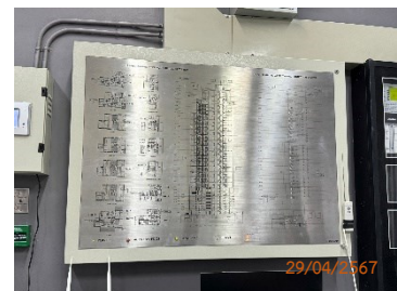
Graphic Annunciator Fire Alarm System
