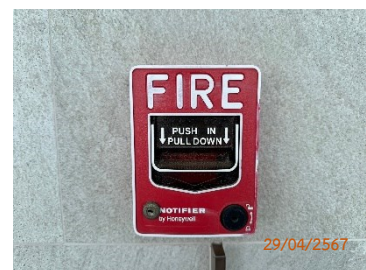
Fire Alarm Manual Station
