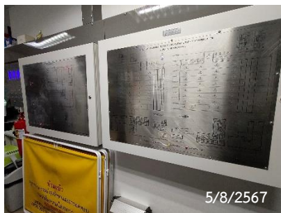
Graphic Annunciator Fire Alarm System
