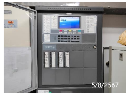
Fire Alarm Control Panel
