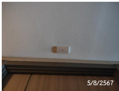
Fire Alarm Indicator Lamp
