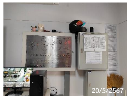
Graphic Annunciator Fire Alarm System
