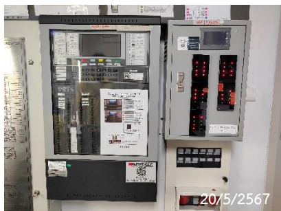
Fire Alarm Control Panel
