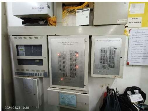
Fire Alarm Control Panel
