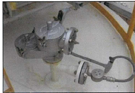
Pressure Vacuum Relief Valve
