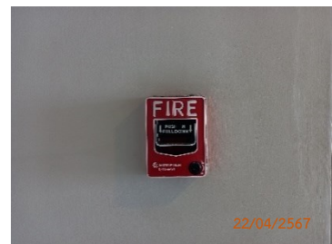
Fire Alarm Manual Station
