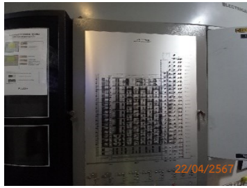
Graphic Annunciator Fire Alarm System
