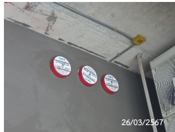
Sprinkler Fire Alarm When Bell Rings
