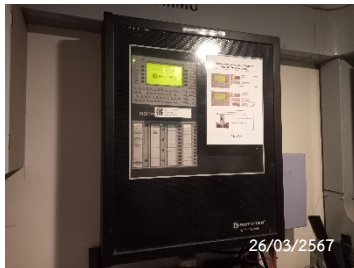
Fire Alarm Control Panel
