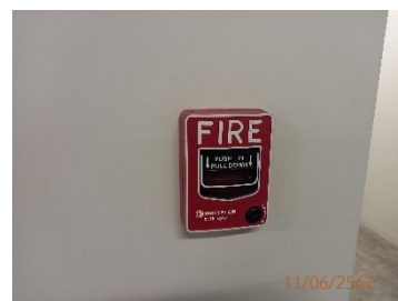
Fire Alarm Manual Station
