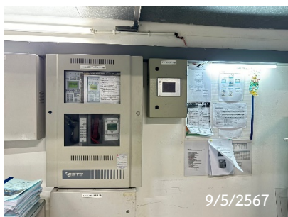
Fire Alarm Control Panel
