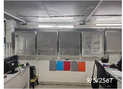
Graphic Annunciator Fire Alarm System
