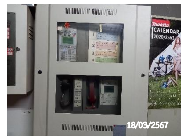
Fire Alarm Control Panel
