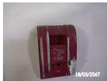
Fire Alarm Manual Station
