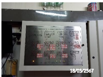
Graphic Annunciator Fire Alarm System
