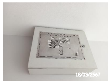
Graphic Annunciator Fire Alarm System
