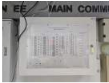
Fire Alarm Control Panel
