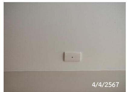
Fire Alarm Indicator Lamp
