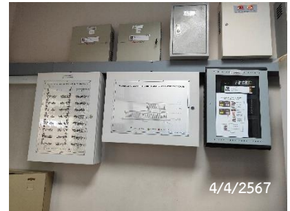
Graphic Annunciator Fire Alarm System
