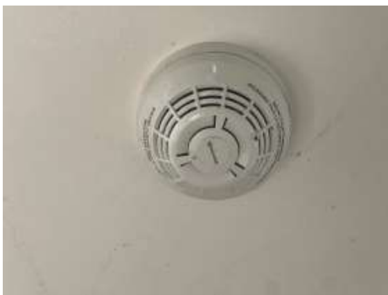
Rate of Rise Heat Detector
