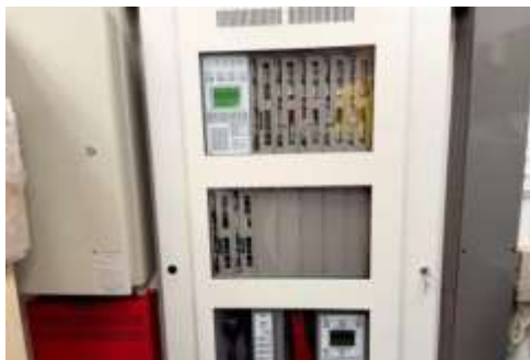
Fire Alarm Control Panel
