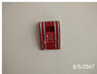
Fire Alarm Manual Station
