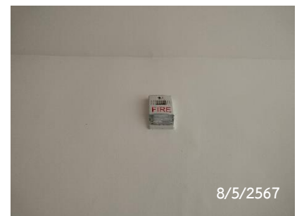
Fire Alarm Horn Strobe
