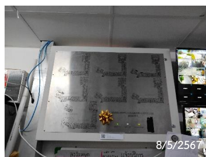
Graphic Annunciator Fire Alarm System
