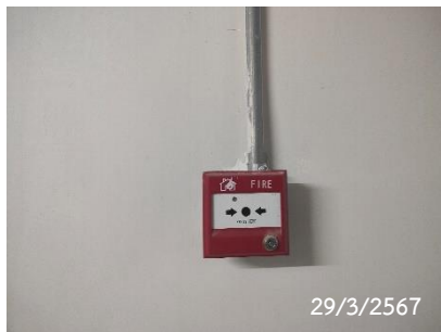
Fire Alarm Manual Station
