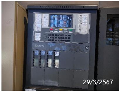
Fire Alarm Control Panel
