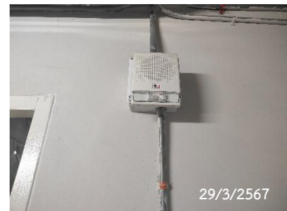
Fire Alarm Horn Strobe
