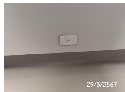
Fire Alarm Indicator Lamp
