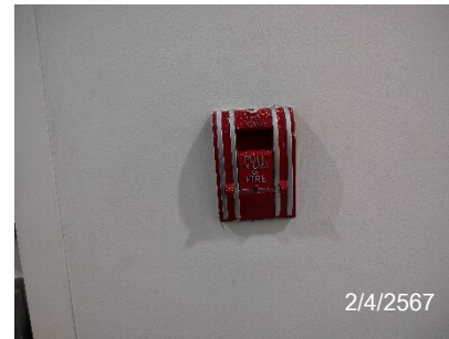
Fire Alarm Manual Station
