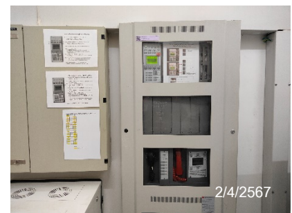
Fire Alarm Control Panel
