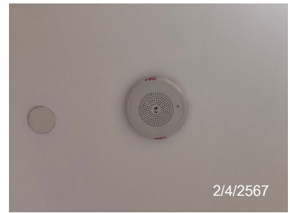
Fire Alarm Horn Strobe
