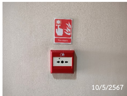
Fire Alarm Manual Station
