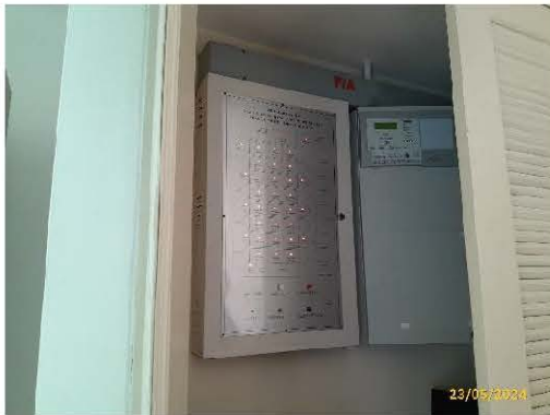
Fire Alarm Control Panel
