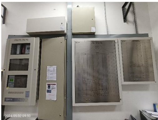
Fire Alarm Control Panel
