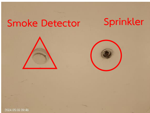
Smoke Detector & Sprinkler
