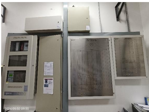
Fire Alarm Control Panel
