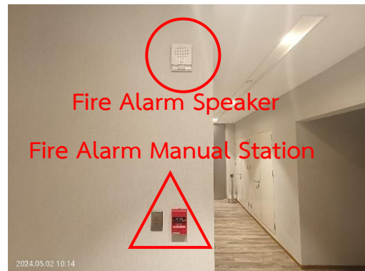
Fire Alarm Speaker & Fire Alarm Manual Station
