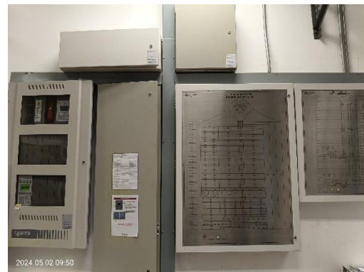
Fire Alarm Control Panel
