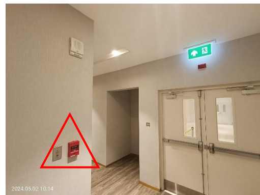
Fire Alarm Manual Station
