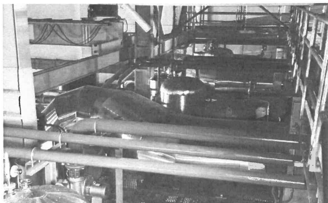
Install insulation and aluminum jacket for duct
