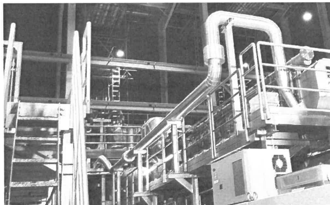
Install insulation and aluminum for oil mist pipe
