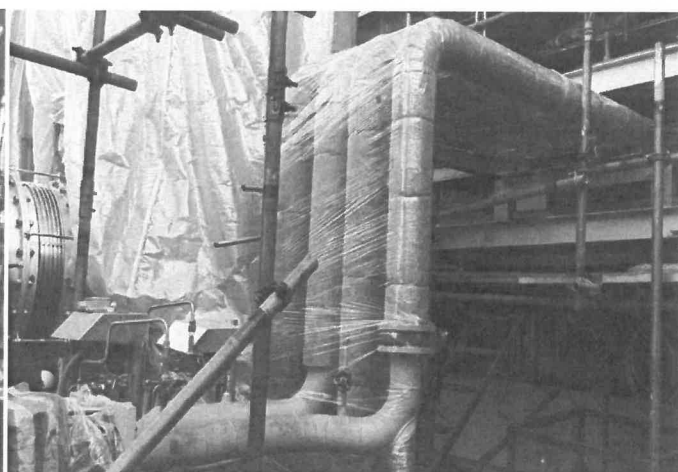
Install Insulation for Cooling Water Pipe
