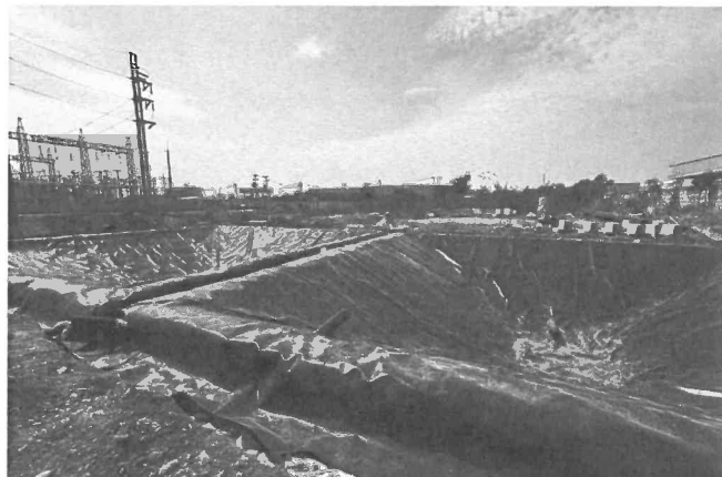
Install HDPE Sheet
