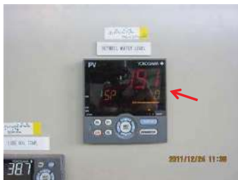
5. Stop make-up water pump at +170mm *Indication color will be red at \geq +170\text{mm} or \leq -170\text{mm}
