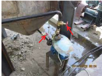
3. Check make-up water pump *Open valves
