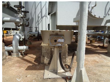
Hydrocarbon Gas Detector
