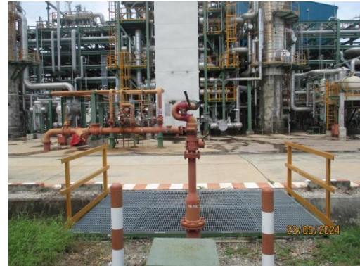
Water Hydrant with Monitor
