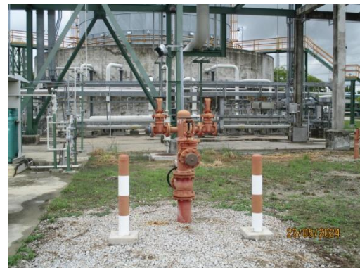
Water Monitor with Remote
