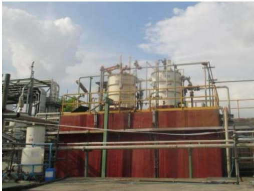
Neutralization Tank
