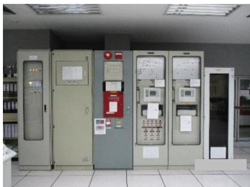
Master Fire Alarm Control Panel
