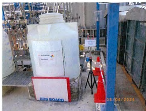
Sodium hydroxide tank (Boiler)
