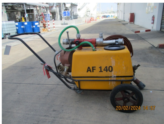
Wheel Foam Chemical Extinguisher
