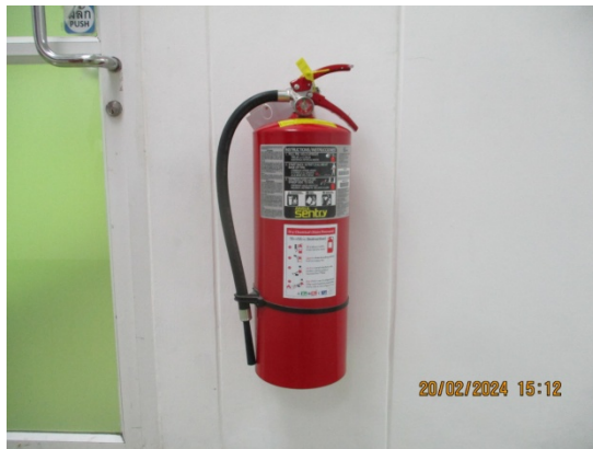
Portable Dry Chemical Extinguisher
