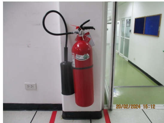
Portable Fire Extinguisher (CO 2 )
