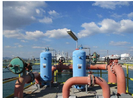
Fire Water Accumulator
