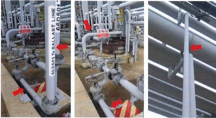
Photo15: 66D501 to ballast line still in good condition observed.
