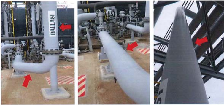
Photo9: 66K302 to ballast line still in good condition observed.
