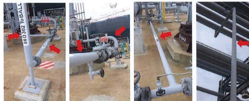
Photo8: 66D302 to ballast line still in good condition observed.
