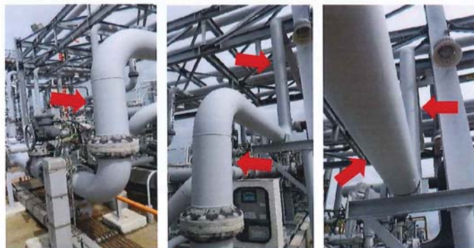
Photo5: 66HV218 to ballast line still in good condition observed.
