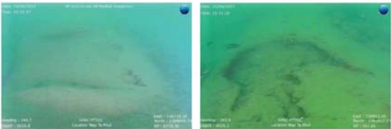
Typical Field Joint Condition - KP8.718
