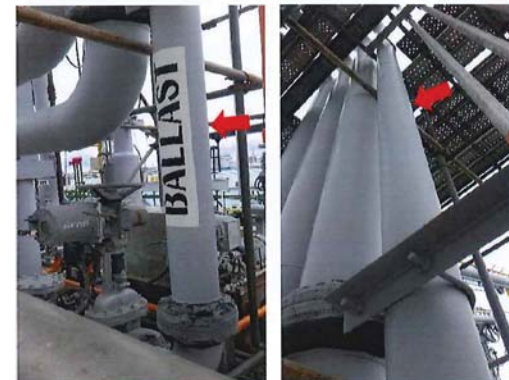
Photo14: 66HV519 to ballast line still in good condition observed.
