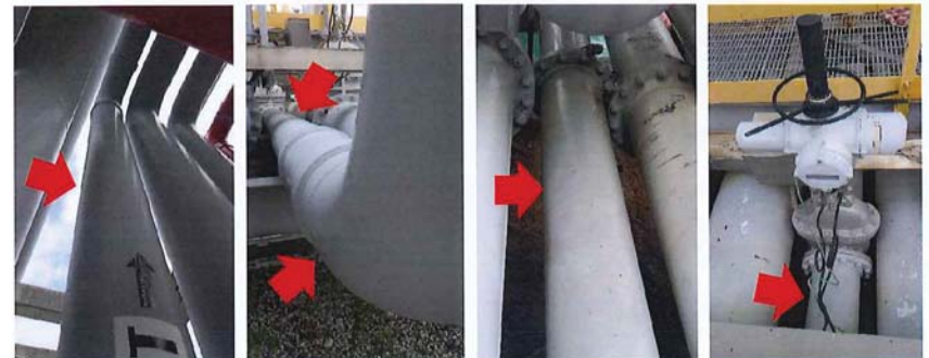
Photo2: Ballast line still in good condition observed.
