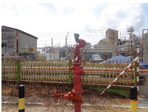
Fire Water Monitor with Foam Induction
