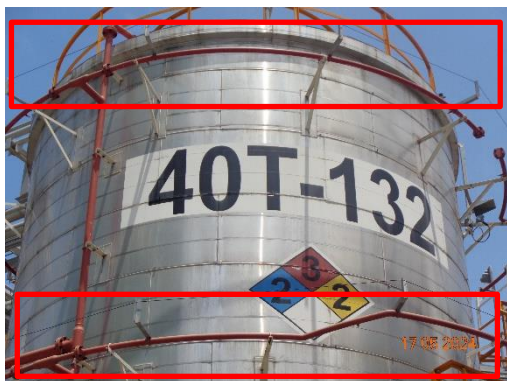
Automatic Water Sprinkler System
