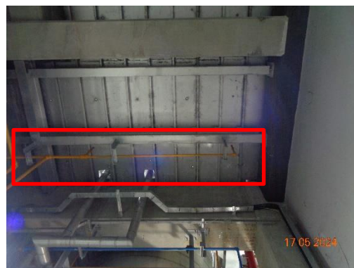
Automatic Foam Sprinkler System
