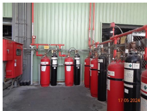
CO 2 Extinguishing Systems
