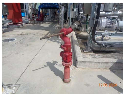
Fire Water Hydrants with Water Monitor
