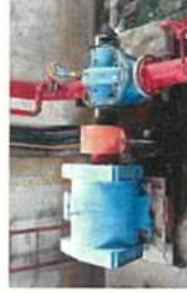
Motor Water Pumps, STP brand, Type TD12D 2969RPM, Head 102, Flow Meter 85 litres / Sec.
