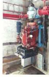
Motor Water Pumps, STP brand, Type TD12D 2969RPM, Head 102, Flow Meter 85 litres / Sec.
