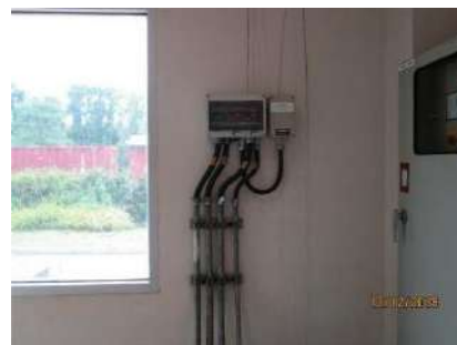
Chlorine Gas Leak Detector
