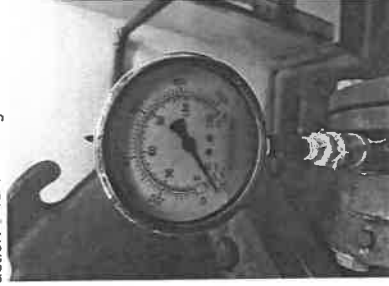
Figure 3.1 Pressure gauge of suction side is damaged.
