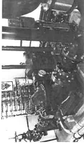
Figure 2.3 Fire pump no.1 (Low Zone)
