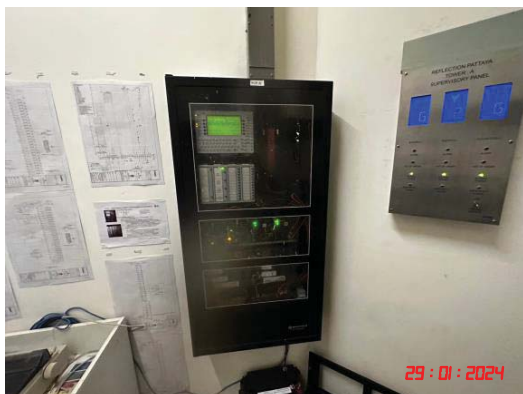
Fire alarm control panel
