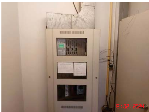
Fire Alarm Control Panel
