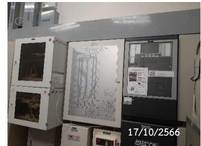
Graphic Annunciator Fire Alarm System
