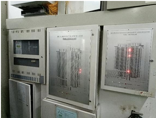
Fire Alarm Control Panel
