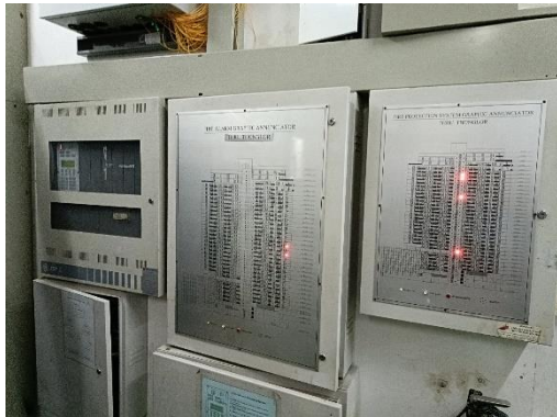
Fire Alarm Control Panel
