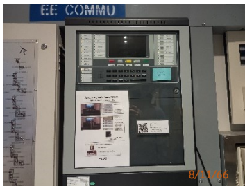
Graphic Annunciator Fire Alarm
