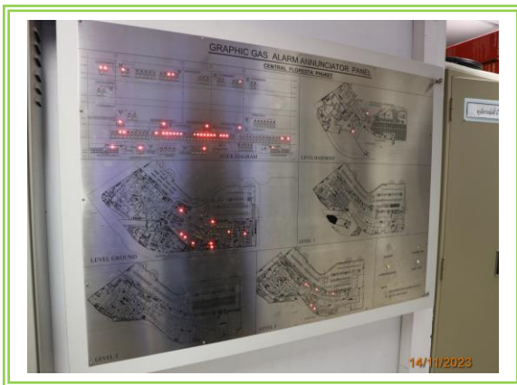
Graphic Annunciator Fire Protection System
