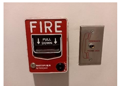
Fire Alarm Manual Station
