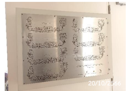
Graphic Annunciator Fire Alarm System
