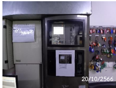
Fire Alarm Control Panel
