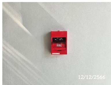
Fire Alarm Manual Station
