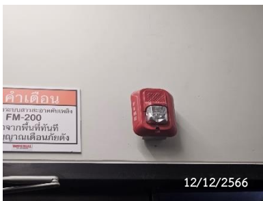
Fire Alarm Horn Strobe
