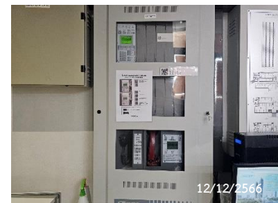
Fire Alarm Control Panel
