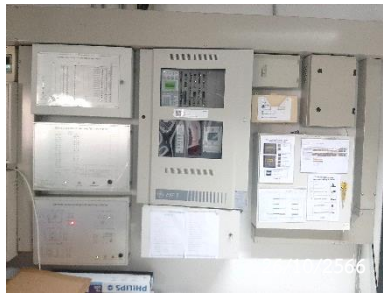
Fire Alarm Control Panel
