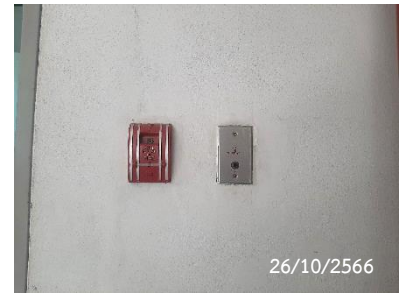
Fire Alarm Manual Station
