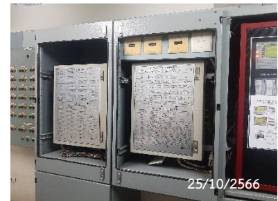
Graphic Annunciator Fire Alarm System
