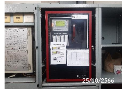
Fire Alarm Control Panel
