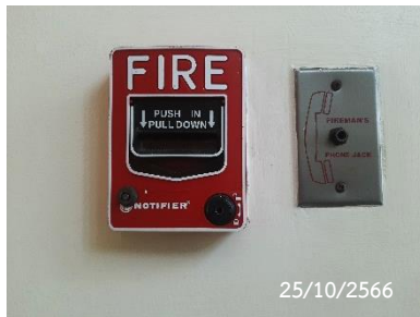
Fire Alarm Manual Station
