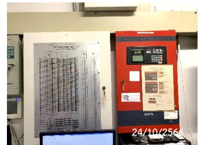
Fire Alarm Control Panel
