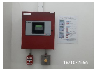
Fire Alarm Control Panel
