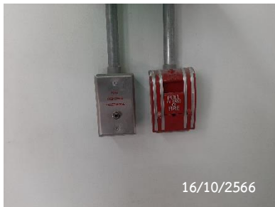
Fire Alarm Manual Station
